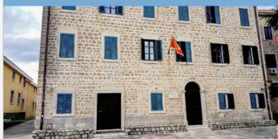
#3 Building of the music school Herceg Novi
